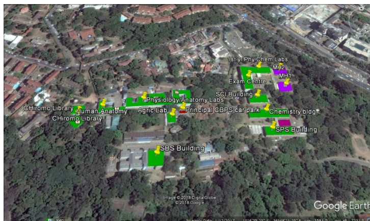
Fig. 1: Chiromo Campus Roof Area with a roof Area of 12,127 m 2 with a 1,819 kWp Generation Potential
